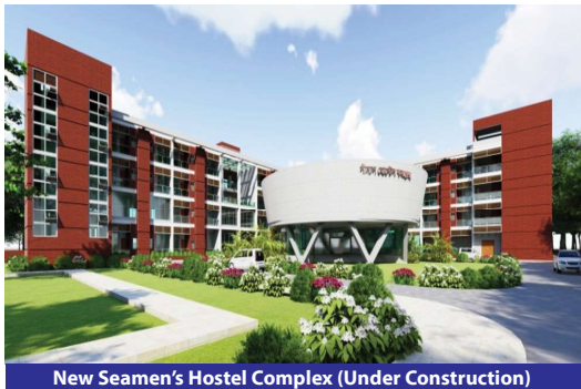
New Seamen's Hostel Complex (Under Construction)
